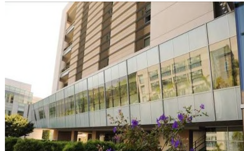
Bridge to/from Brawerman Center
