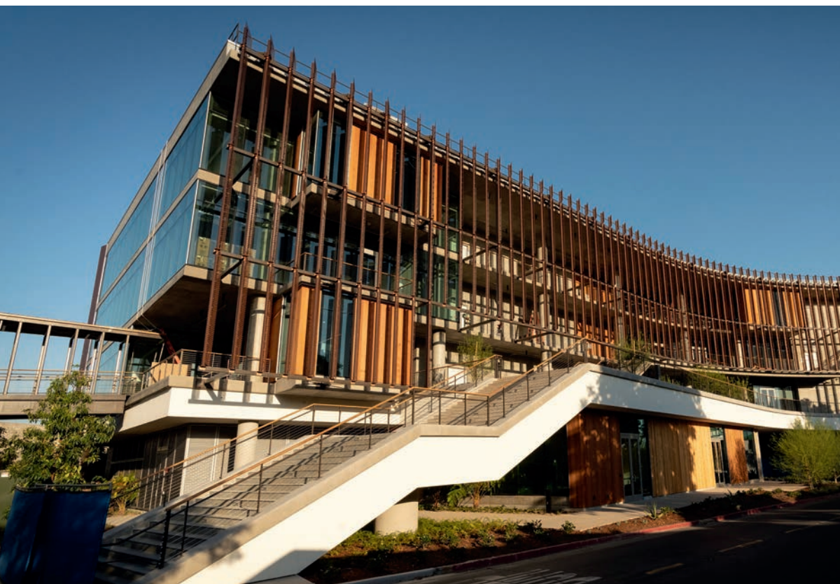
City of Hope's $1 billion main campus expansion continues during the pandemic. Pictured is the new four-story Medical and Administrative Leadership Pavilion.
